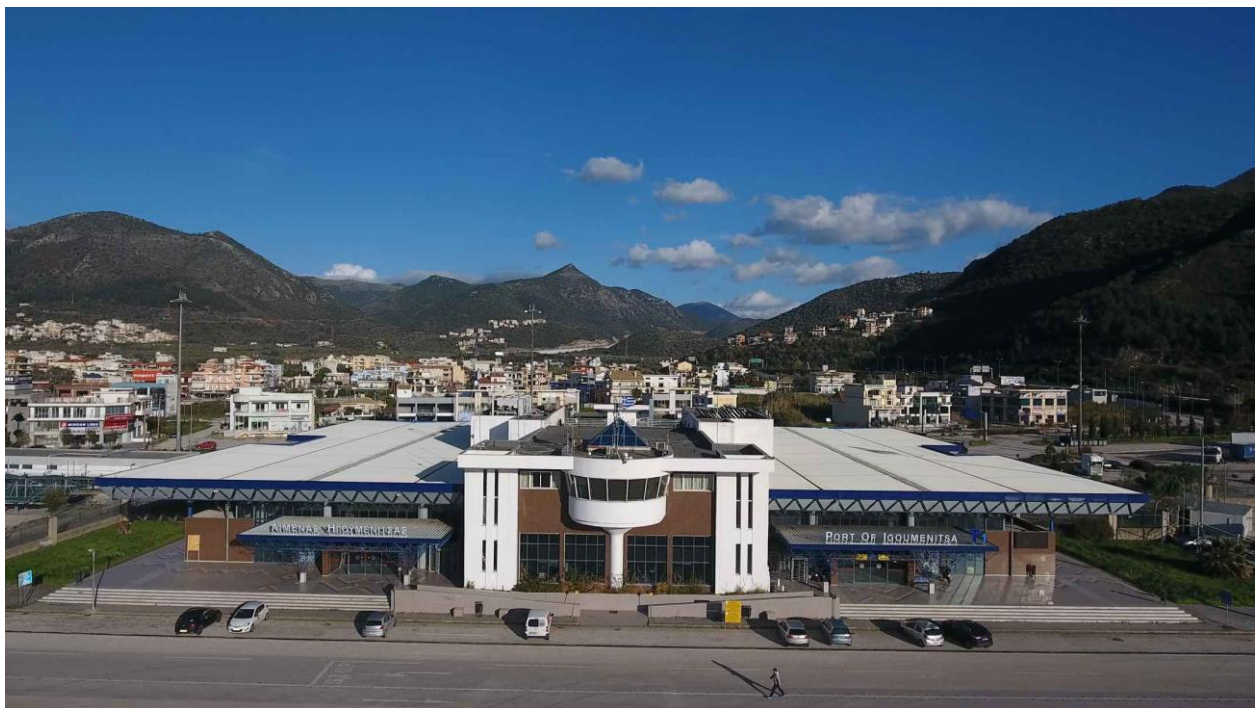
Igoumenitsa Port Facilities
