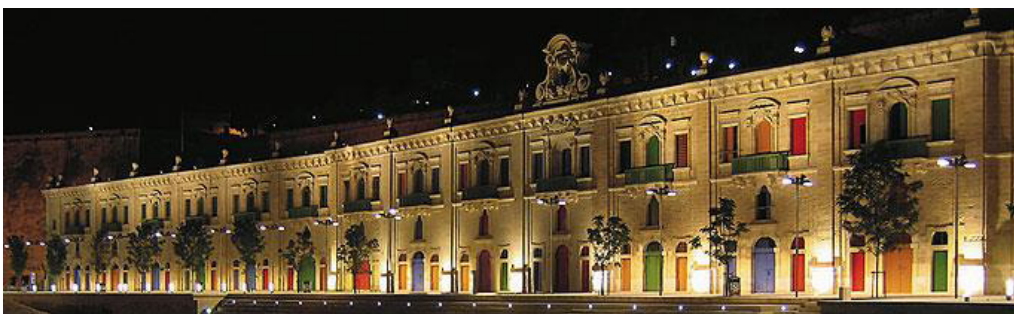
Figure 3: The Restored Façade of Pinto Wharf, Floriana known as Valletta Waterfront
