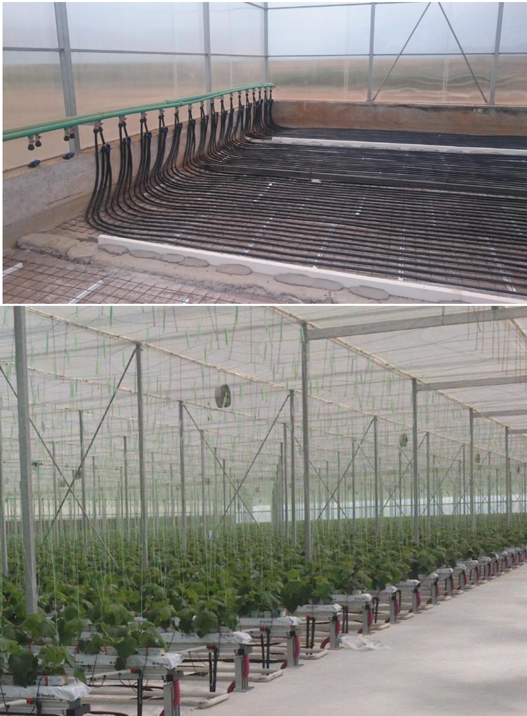
Figure 15. Surface heating system in u-bond design.
