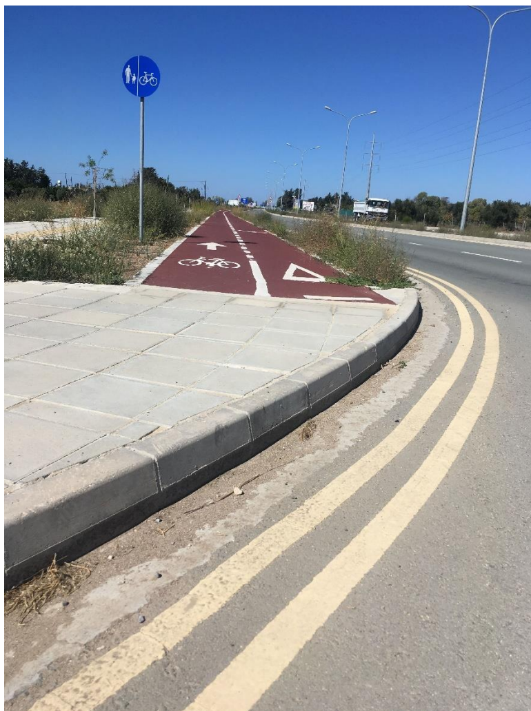
High kerb at the edge of a segregated cycle path in Pafos
