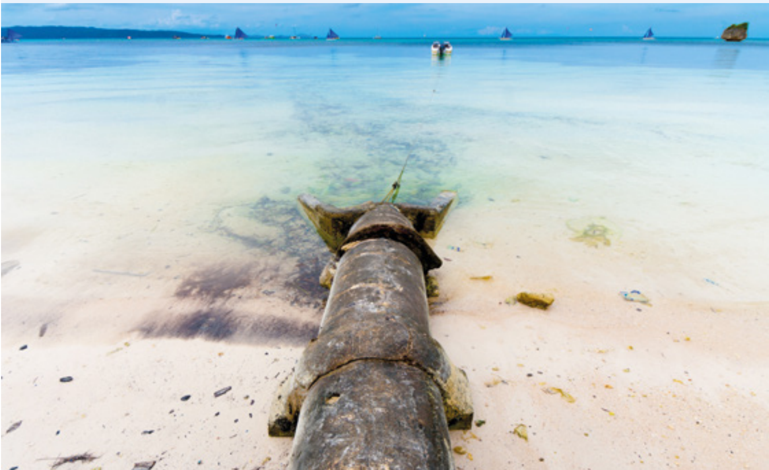
Fig. C: Wastewater pipe ending directly in the sea.
