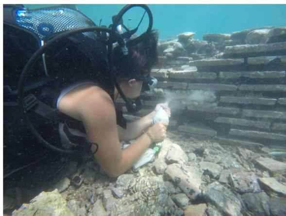
Fig. 9. Filling of hinges on a brick wall of the Roman villa by the Ephorate of Underwater Antiquities in collaboration with ISCR. Summer 2017. (Photo by Gabriele Gomez De Ayala, copyright ISCR).
