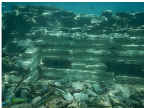
Fig. 10. Façade of brick wall of the Roman villa after the filling of hinges. (Photo by Gabriele Gomez De Ayala, copyright ISCR)
