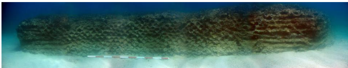
Fig. 3 Structures of the northern pier in a concrete structure covered with an onsite facing of which the trace remains. Photos G. Colucci.
