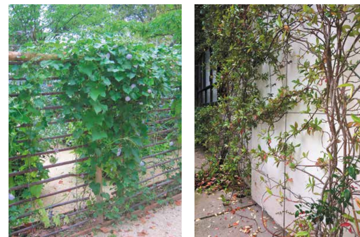
Example of a structure offset from a wall by 10cm with taut stainless-steel cable (Chinese Jasmine).
