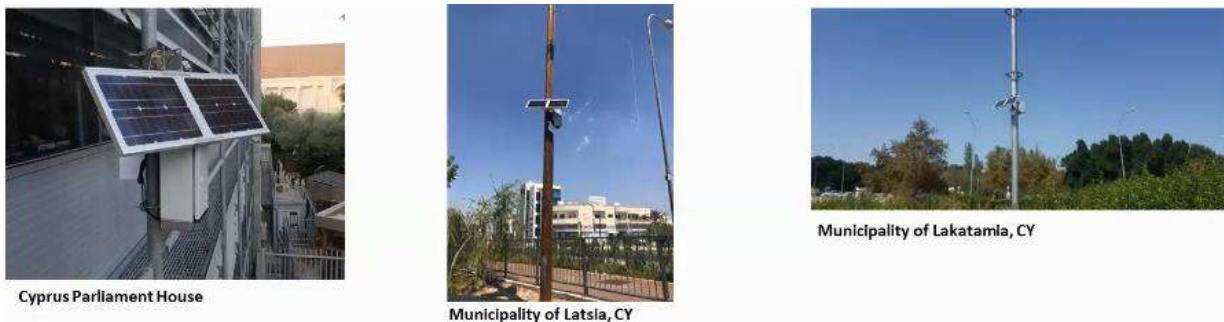
Figure 3: Indicative images of the AIRTHINGS project
