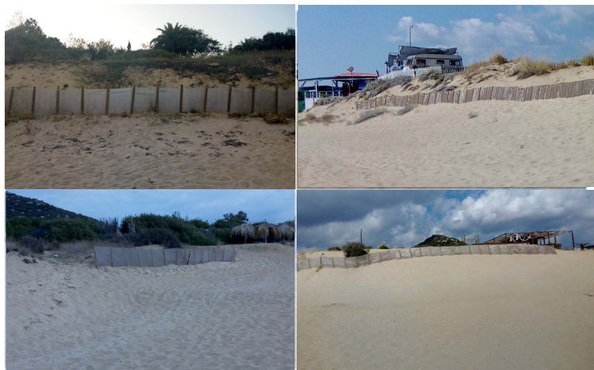
Figure 2. Sand fences for coastal restoration installed in Ammolofi, Greece.
