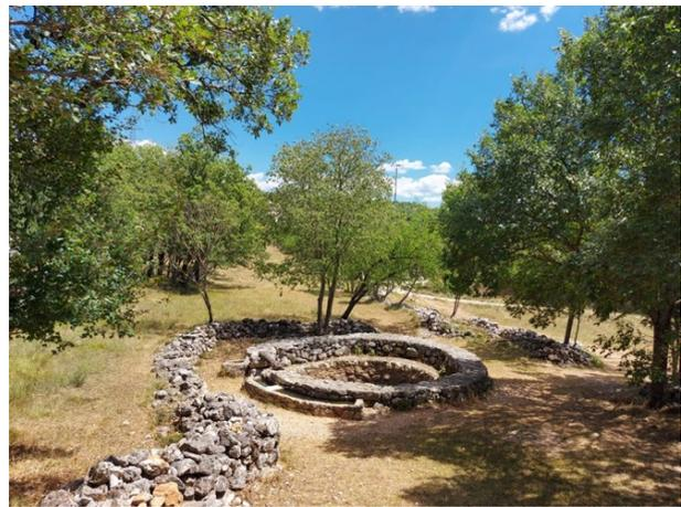
The buildings are built of lime-bound stone, while the stone fences are built using the drywall technique, which has been recognized and protected by UNESCO on the World Intangible
