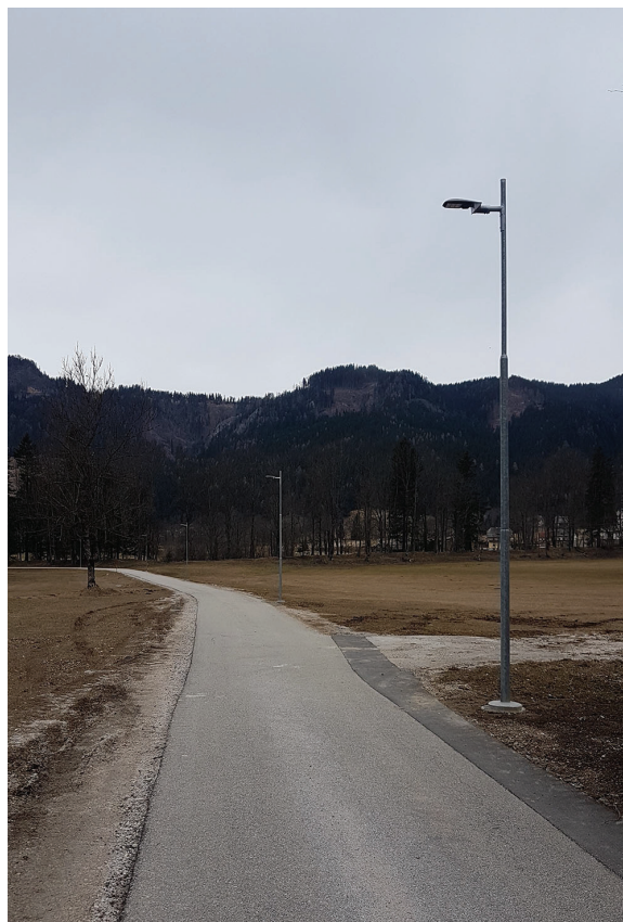
Figure 7: new luminaires on combined poles in Jezersko
