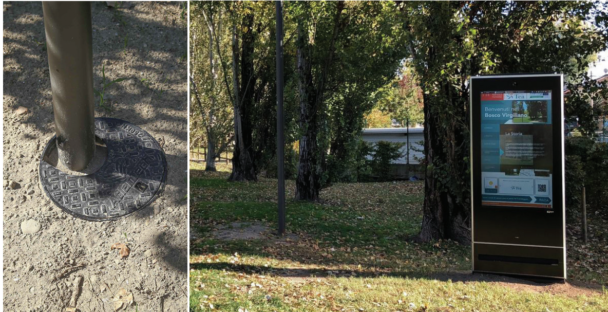
"Screw" Foundations & Multimedia Totem.
