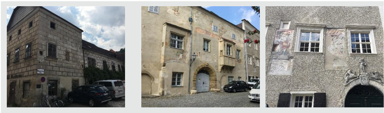
Figure 20. Buildings' facades with adornment and sgraffito articulation.
