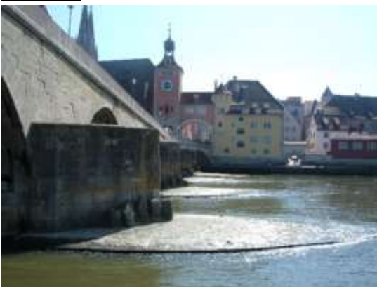
Example of historic protection of bridge piers against undermining (Regensburg)
