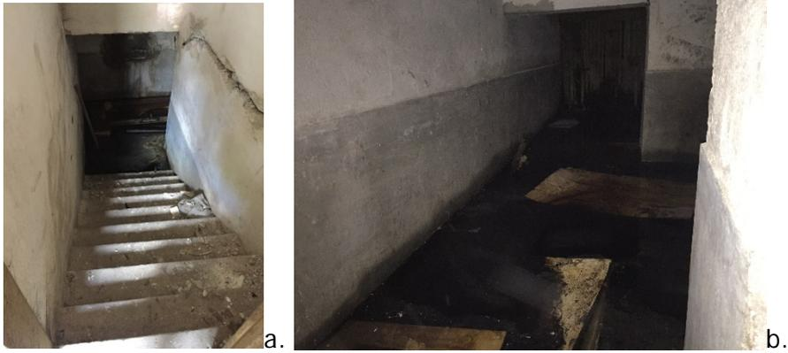
Figure 4. 7. Images a. and b.: Completely flooded basement floor of the building.
