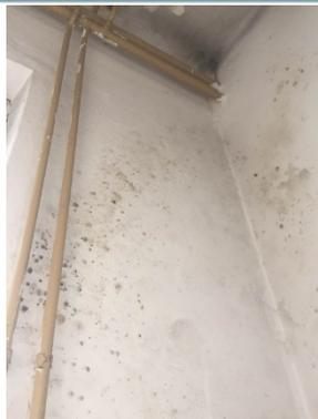
Figure 4. 18. Presence of mildew on outer walls due to leaking façade
