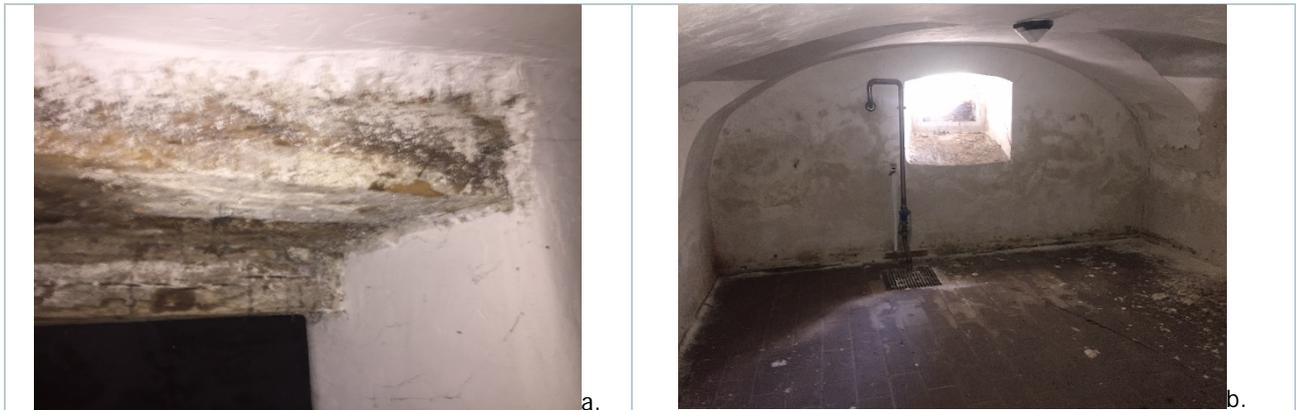
Figure 4. 23. Images a. and b: High volume of rainwater and groundwater in the basement and deterioration of walls
