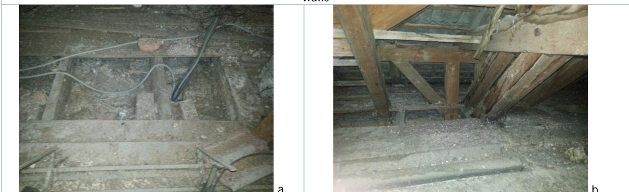
Figure 4. 37. Images a. and b.: Visible leakage of the existing roof coverings and damage on the wooden roof supporting structure and structure between floors
