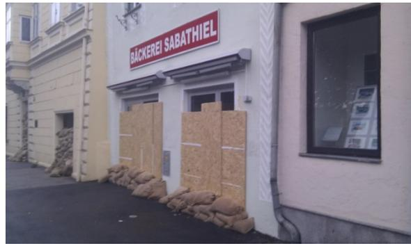
Figure 5. 10. Flood defense systems build up for local shops-Flood Stein 2013.
