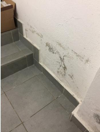
*Figure 4. 5. Visible damp on inner plaster*
