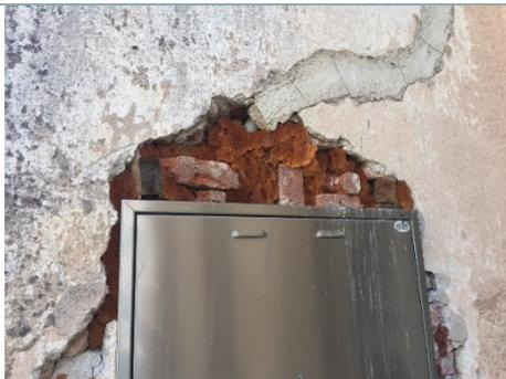
Figure 4. 15. Inappropriate execution of installations on the façade - possibility of leaking
