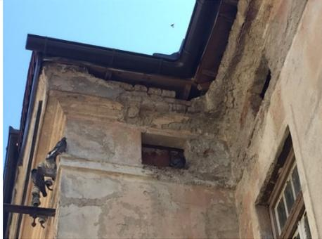
Figure 4. 13. Falling plaster and visible leaking façade
