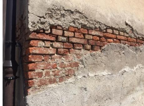
Figure 4. 14. Falling plaster and visible leaking façade
