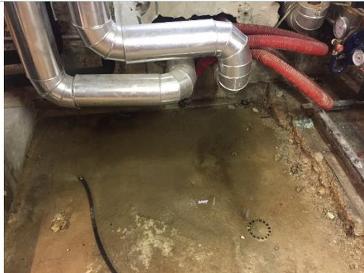
Figure 4. 27. Groundwater in the basement
