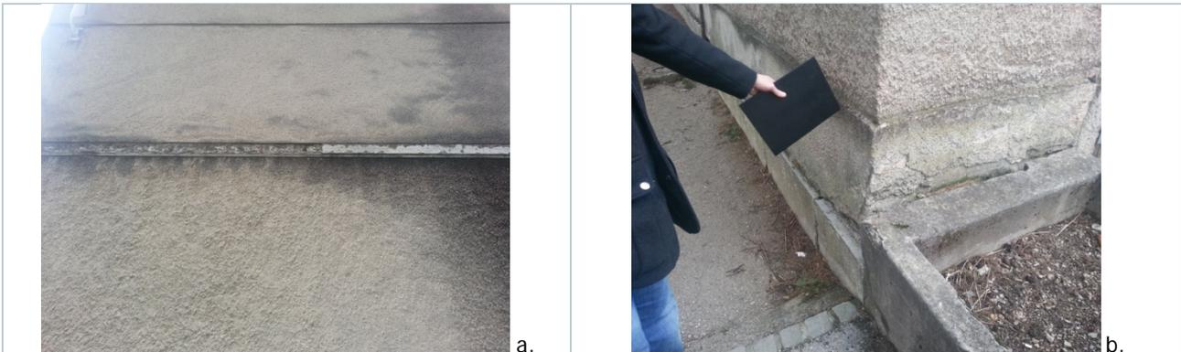
Figure 4. 34. Images a. and b.: Falling plaster and visible leaking façade
