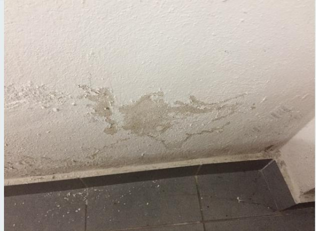
*Figure 4. 6. Visible damp on inner plaster.*
