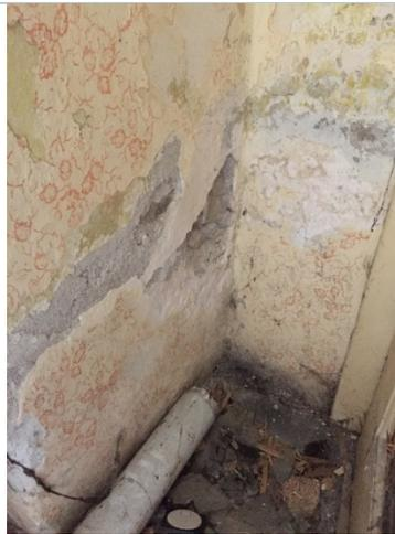
Figure 4. 8. Mildew on outer walls due to water leaking through façade and capillary absorption through non-insulated foundations of the building.
