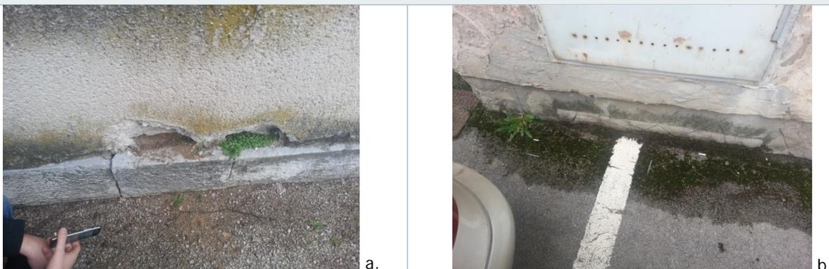
Figure 4. 33. Images a. and b.: Falling plaster and visible leaking façade
