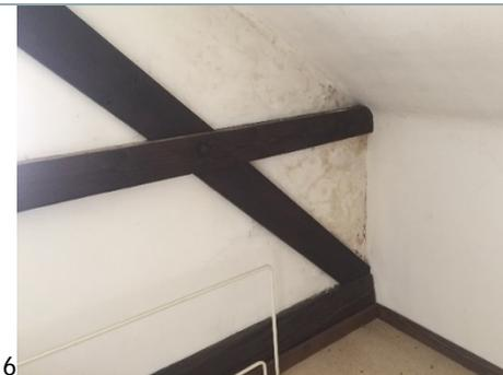
Figure 4. 16. Visible leaking in the mansard due to inappropriate execution of the roof and wear and tear of structure
