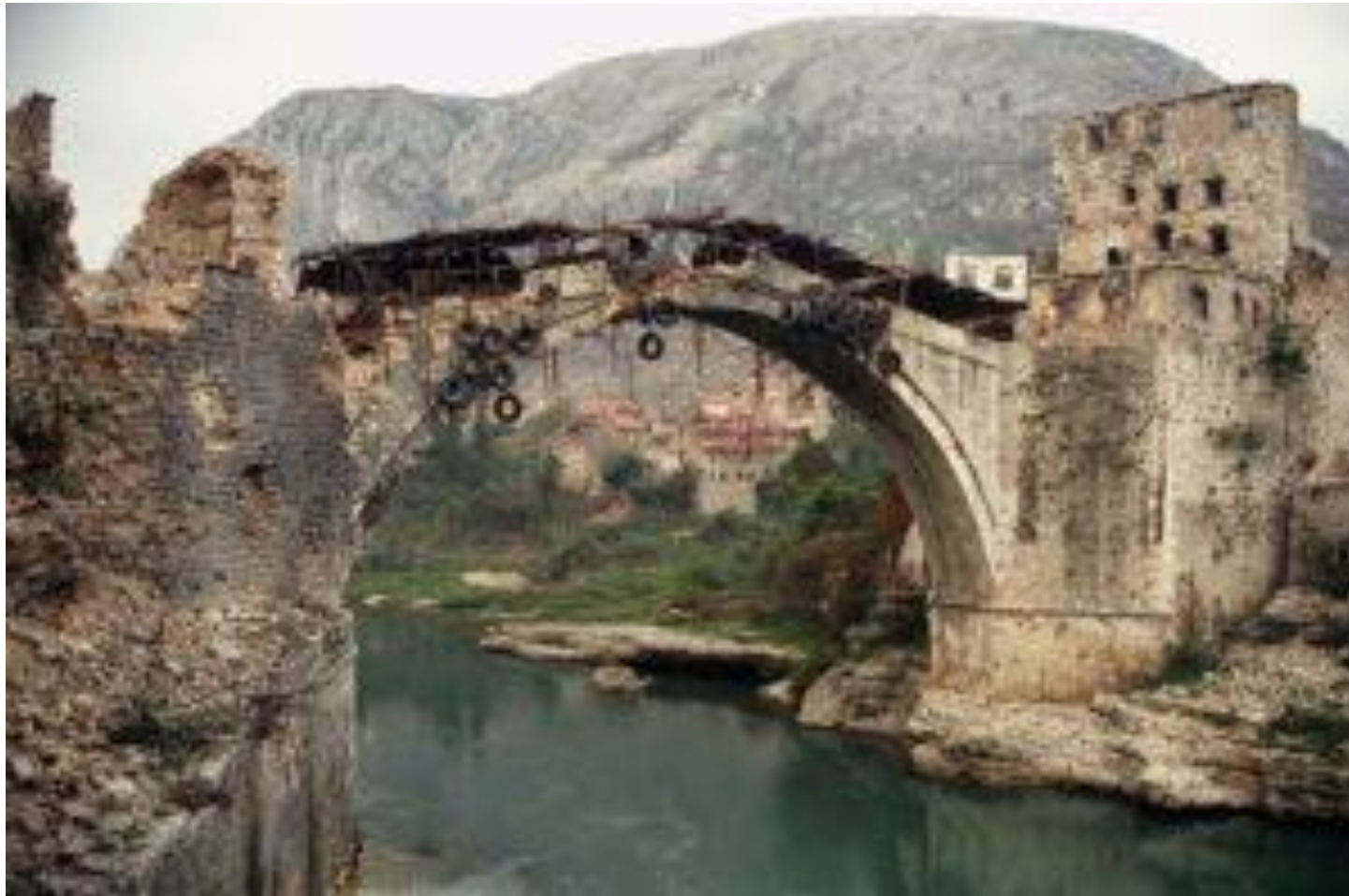
Demolition of the bridge of Mostar, 1993
