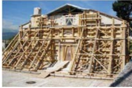
Temporary Shoring in Santa Giusta, L'Aquila
