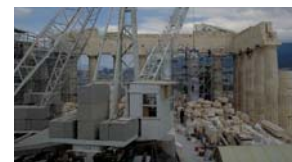
Restoration works on the Parthenon
