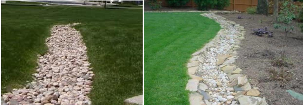
Figure 27. Infiltrating trenches (source: RBMP, Urban rainwater management guide, 2015)
