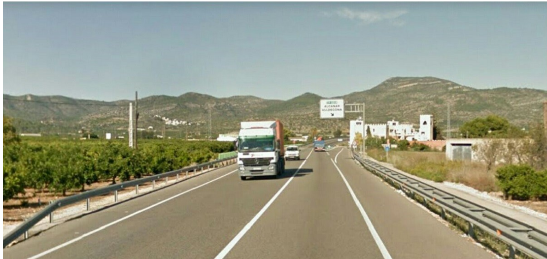
Figure 2.3: N-340 road crossing Alcanar municipality 21
