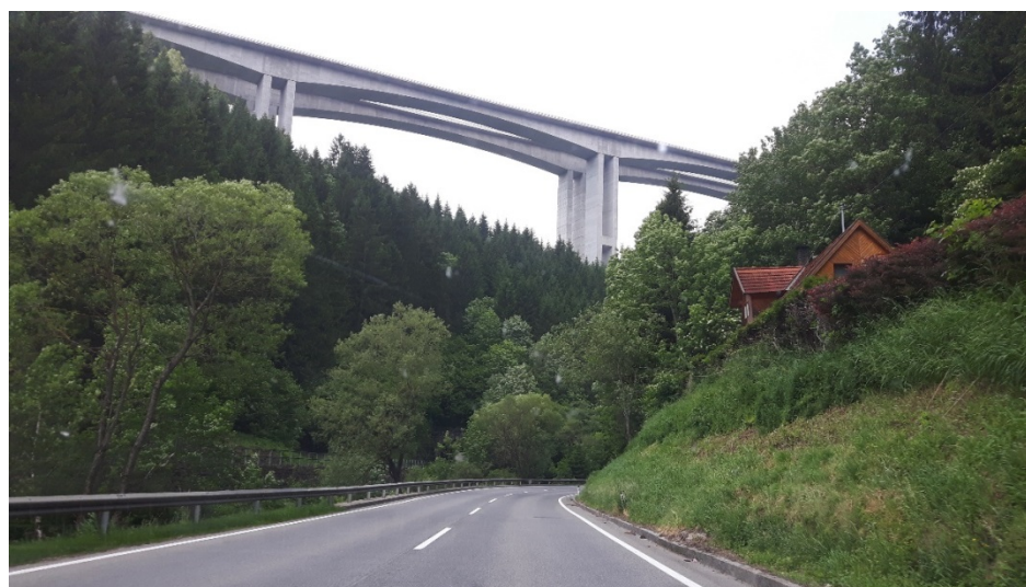
Figure 2.3: Highway bridge in the case study area 10
