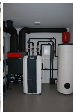
Figure 3: Heat pump - installation is completed
