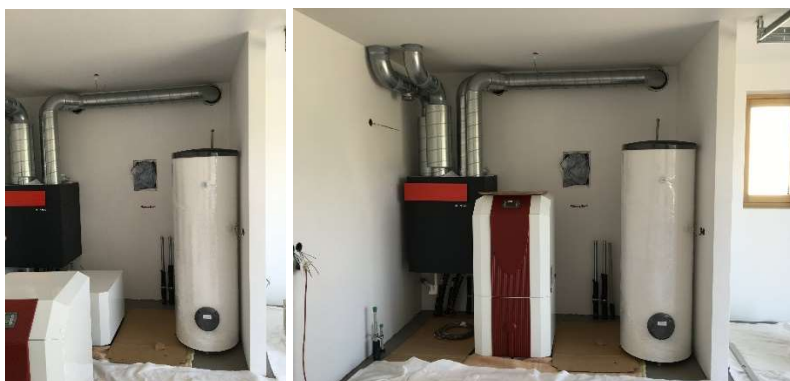
Figure 1-2: Installing a heat pump and ventilation with recuperation
