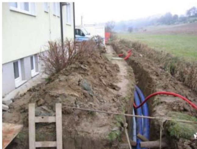
Figure 1-3: Installing of the biomass district heating, source: http://alfalaval.si/novice/29/dolb_kuzma/
