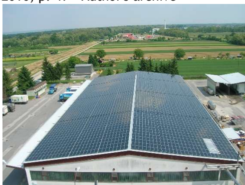
Figure 2: Roof with solar power plant - warehouse plant, April 2011
