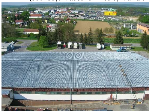
Figure 1: Starting the installation of a solar power plant, April 2011
