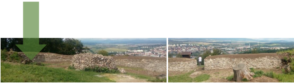
Figure 13 Restoration of the ramparts of Castle Pustý Hrad
