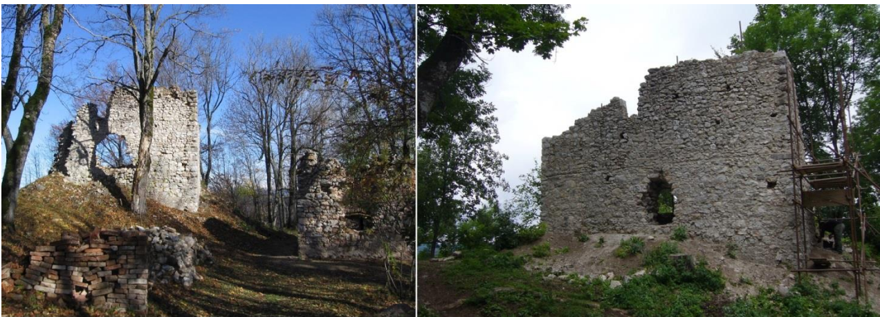
Figure 15 Restoration of the main tower of Castle Muráň
