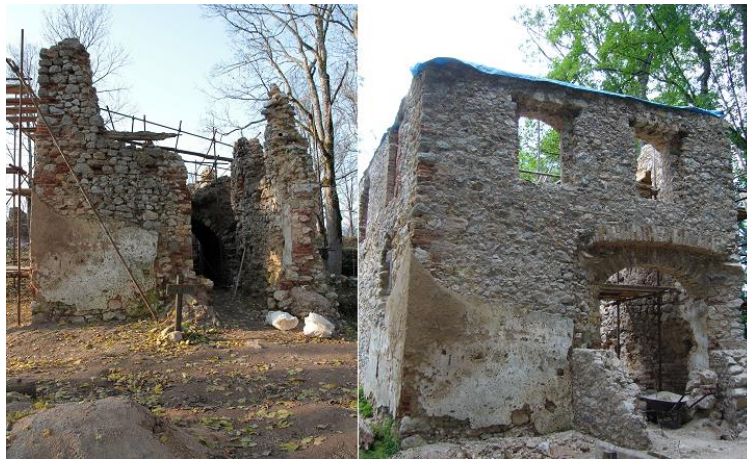
Figure 14 Restoration of captain's residence at Castle Muráň
