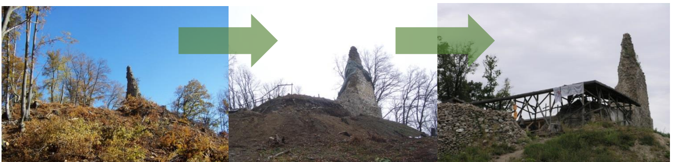
Figure 12 Restoration of the main tower of Castle Pustý Hrad
