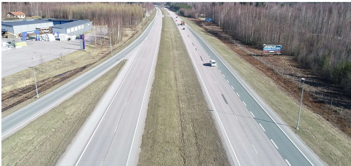
Figure 21. The infrastructure of the Tampere-Helsinki highway was carefully analysed from a platooning perspective. (Picture: Ramboll)
