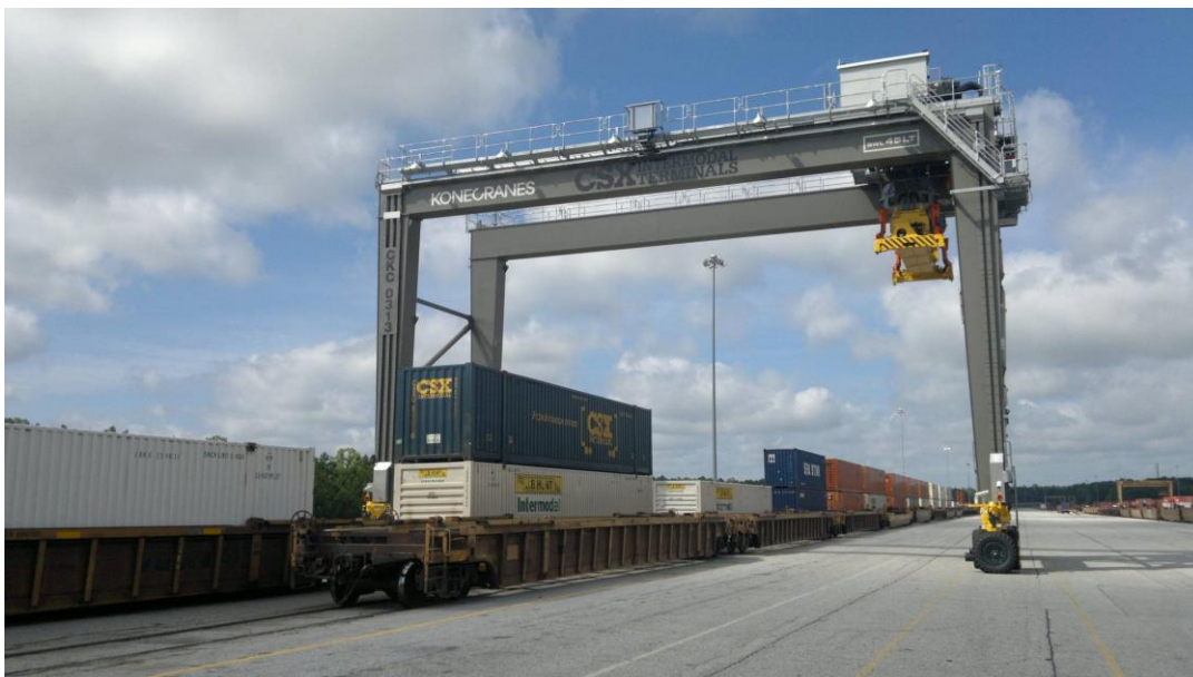
Figure 20. Rubber Tired Gantry Crane (RTG) Source: forkliftaction.com
