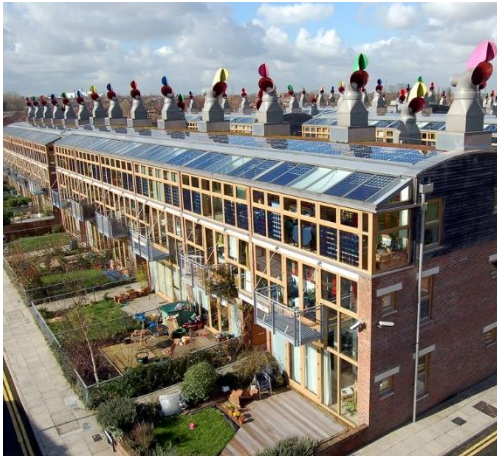
Figure 38. Roof-integrated PV installation. [Photo by telex4 on Foter.com / CC BY]
