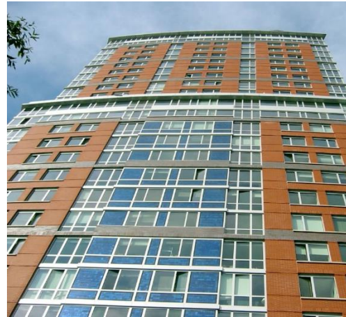
Figure 39. Window-integrated PV installation. [Photo by Payton Chung on Foter.com / CC BY]
