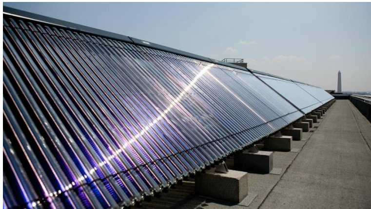
Solar collectors (evacuated tube) on top of a building with the appropriate inclination
