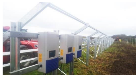
Figure 34. Some inverters in a PV installation in construction. [Source: Source: Ecofutur Solar Company]
