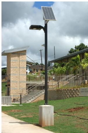
Figure 42. PV installation on a streetlight. [Photo by NAVFAC on Foter.com / CC BY]
