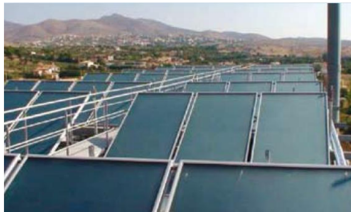
Flat plate collector arrays on top a building roof
