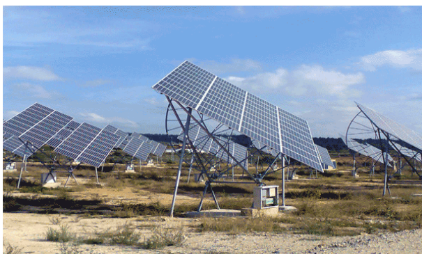
Figure 48. A tracking PV installation. [Source: Ecofutur Solar Company]
