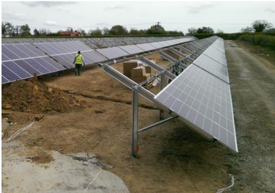
Figure 47. A PV installation made with fixed structure. [Source: Ecofutur Solar Company]
