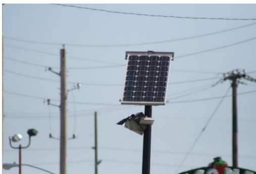
Figure 40. A PV installation on a traffic sign. [Photo by Les_Stockton on Foter.com / CC BY-NC-S]
