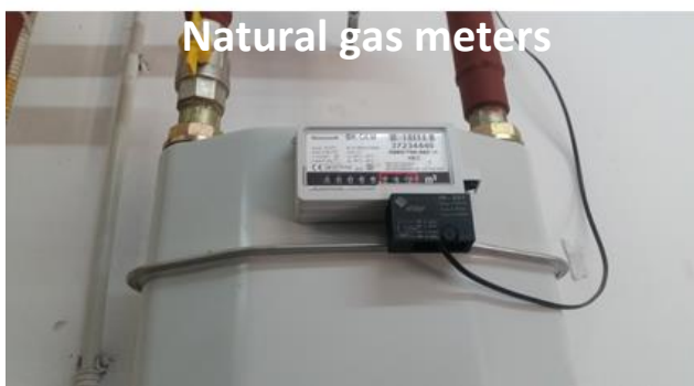
Figure 1: Smart metering hardware implementation. Source: REAN
