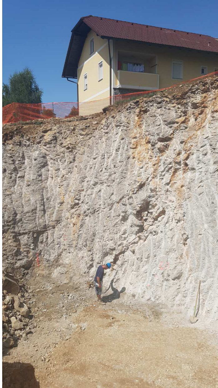
Figure 2: Excavation for wood chips storage
