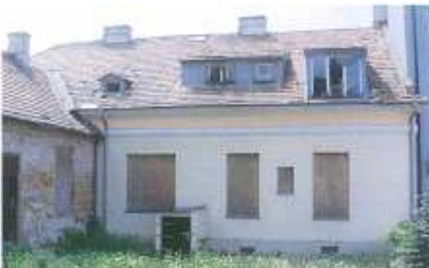
Building view (state before demolition)
