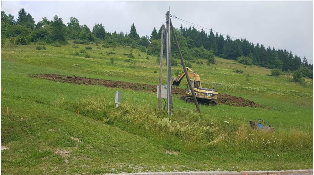
Figure 5: Beginning of the construction works – 6.7.2017
