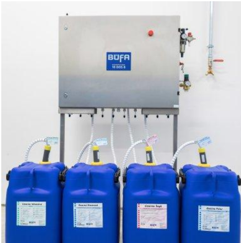
Fig. No. 10: Peristaltic dosing system of Büfa company (www.buefa.ge, 2019) 18)
