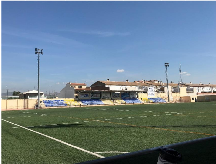
Figure 2. Floodlights at the Huétor Tájar municipal football pitch.
