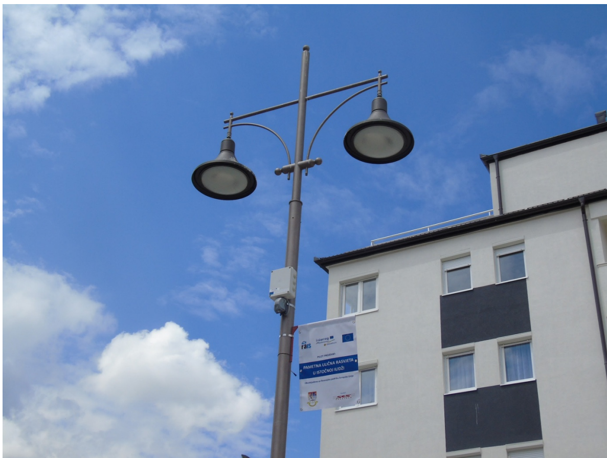
Figure 3.7: On-Site Implementation on Conventional luminaries with HPS bulbs
