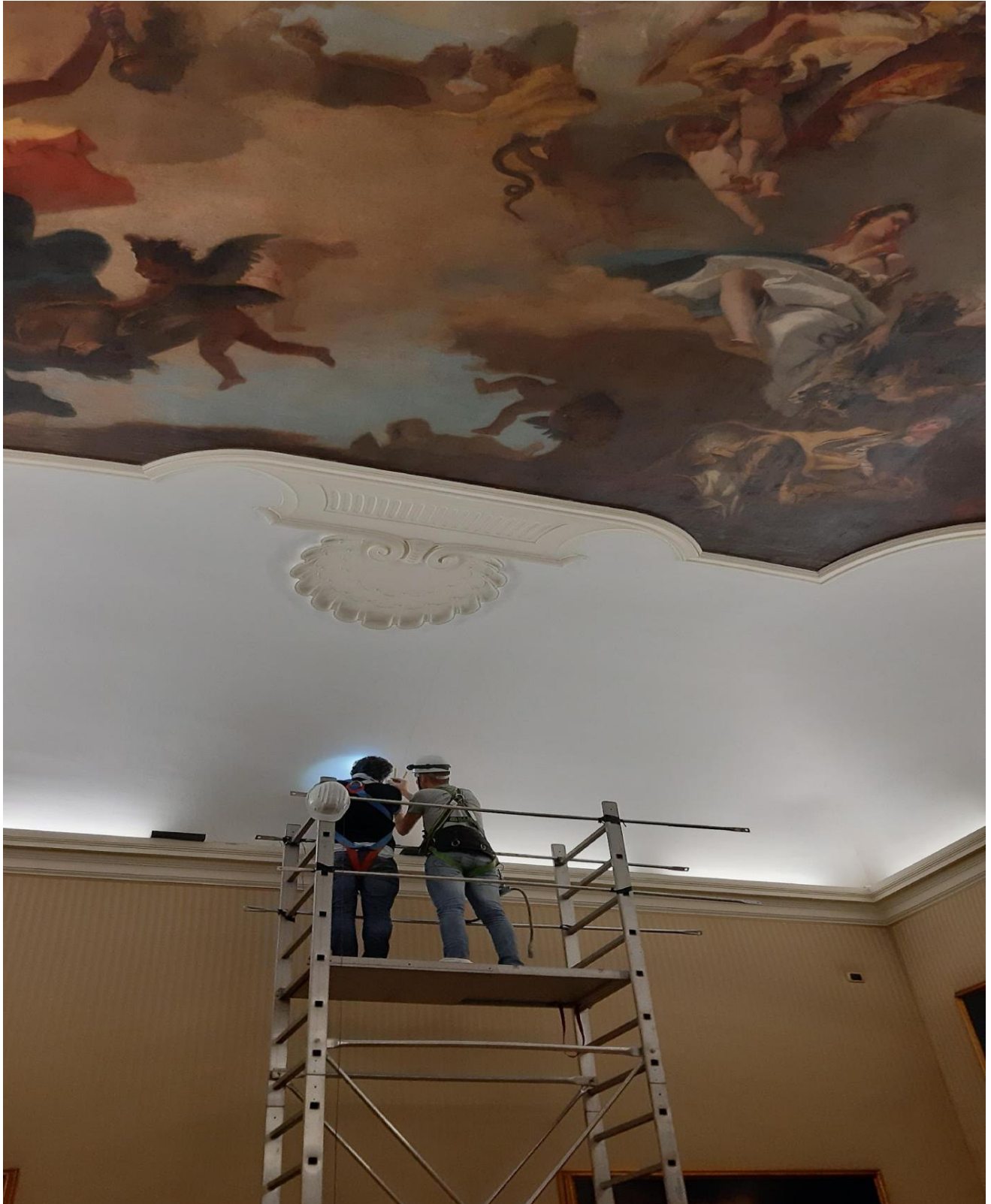
Figure 6 Installation of fiber optic
