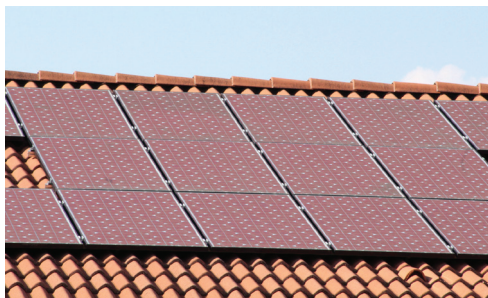
Figura 10: Photovoltaic plant with red panels to decrease the landscape impact (source: www.effettonido.it )
