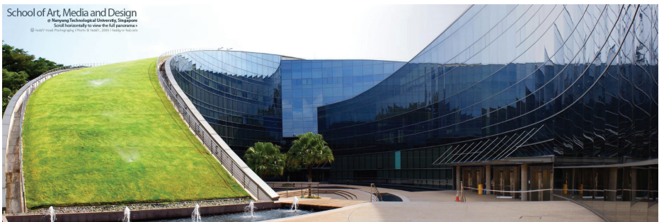
Picture 7: A green roof, example of mitigation and adaptation (source: teddy-rised via Foter.com CC BY-NC-ND)
