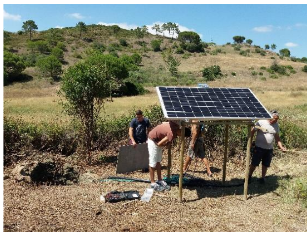
Picture 2– Installation of solar panel on a well
