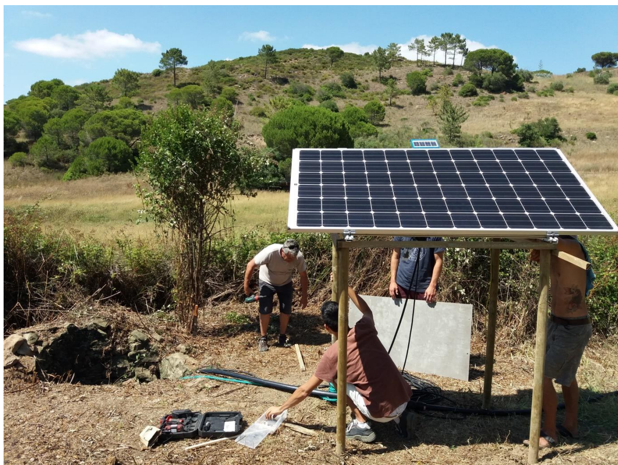
Picture 1 – Installation of solar panel on a well
