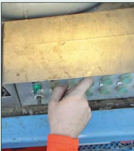
All the manual controls, pumps and indicators etc. are located in the machine room to the front of the unit where an integrated sample point is situated. The purpose of the sample point is to allow the operator to monitor the flocculated sludge during the pumping process.
