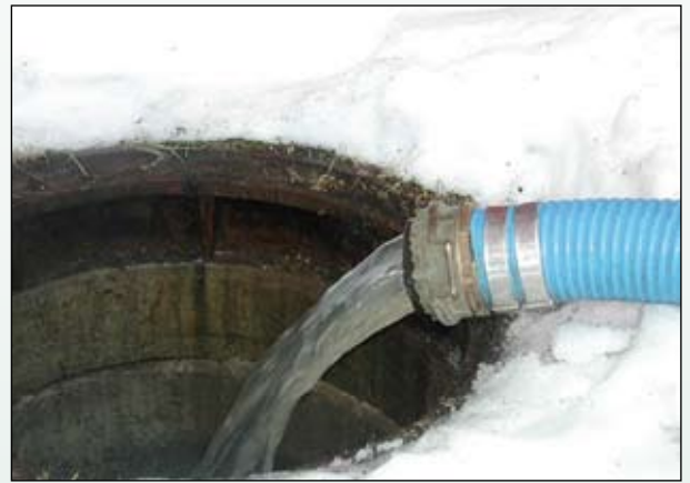
The emptied tanks are refilled with the cleansed water via the KSA.
