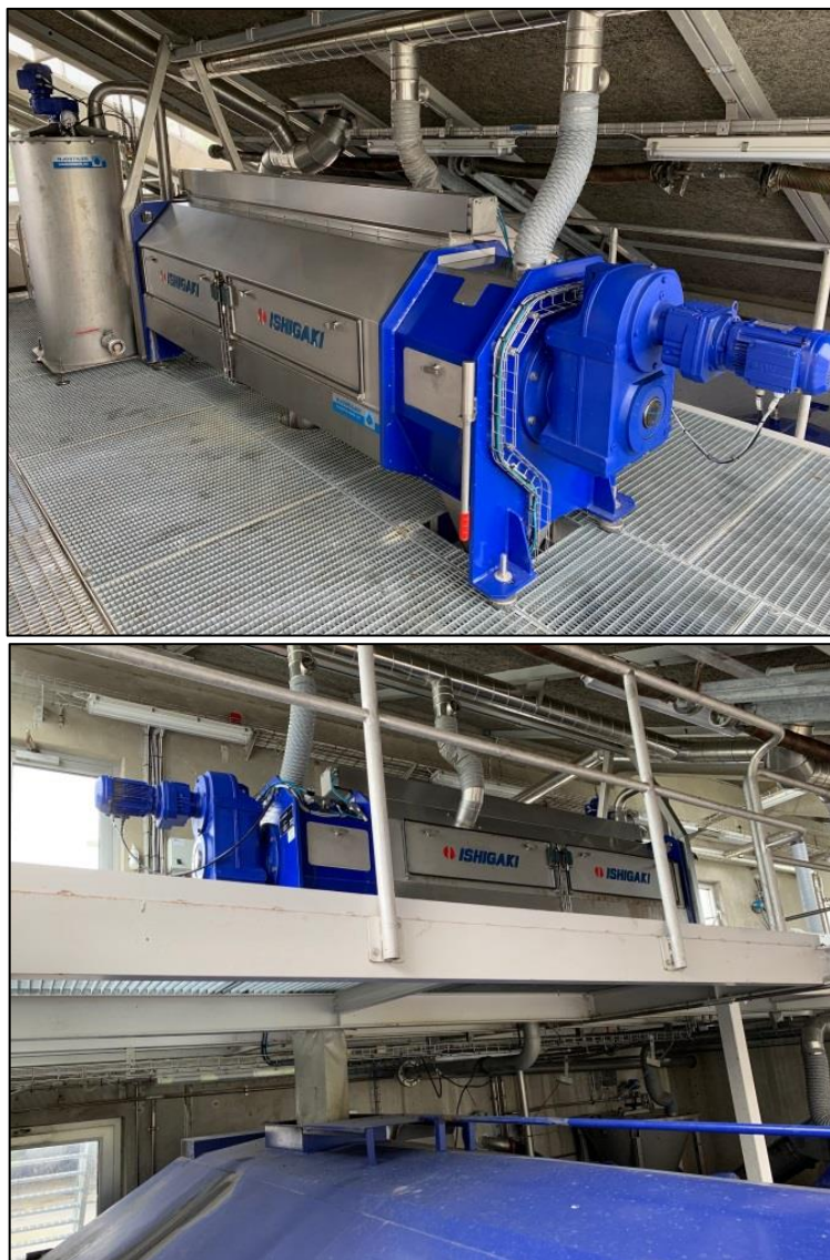
Fig. 3 Screw press for sludge dewatering at Nexø WWTP, Bornholm
