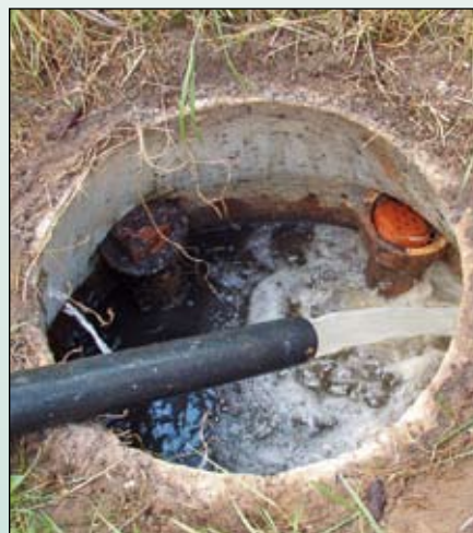
While the sludge is being pumped to the dewatering chamber the operator can return the cleansed water back to its source, this keeps the process time to a bare minimum, just one of the many practical functions which makes the KSA easy and efficient to operate.
