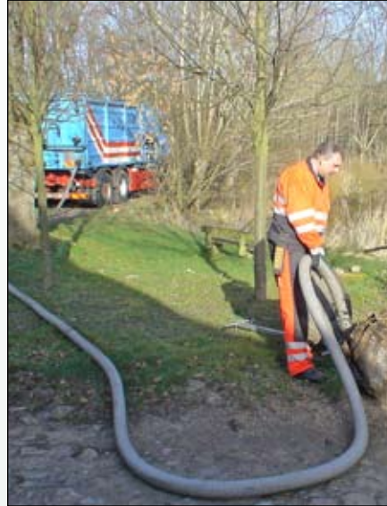
The sludge is taken up into the vacuum tank exactly the same way as you would by a traditional jet-vac or tanker.
