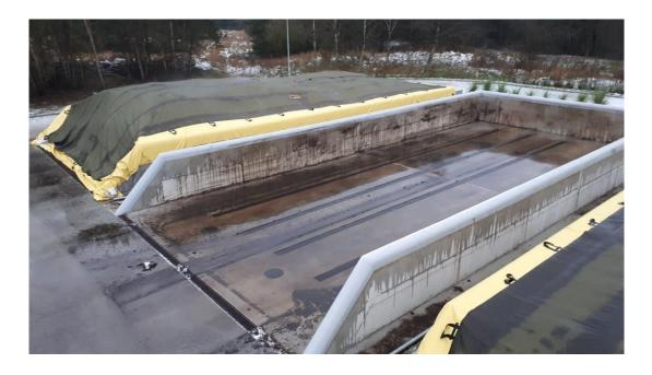
Picture 5. Floor aeration system and drainage channels.
