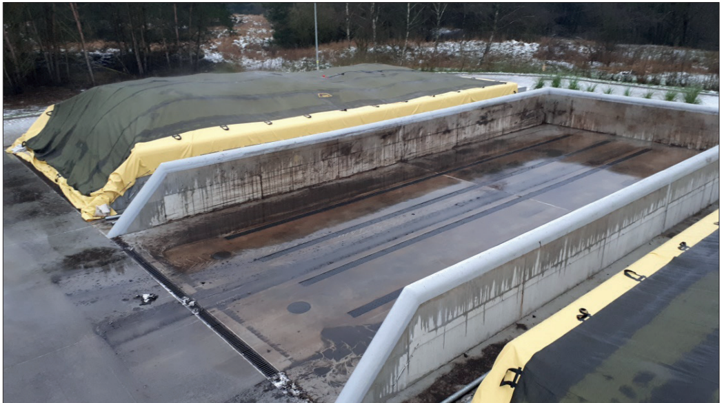
Picture 4. Composting plant with forced aeration.
