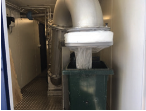
Figure 3. Roto-sieve and wash press
