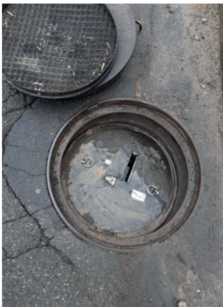
Fig. 13. Measuring device installed in a sanitary sewer chamber
