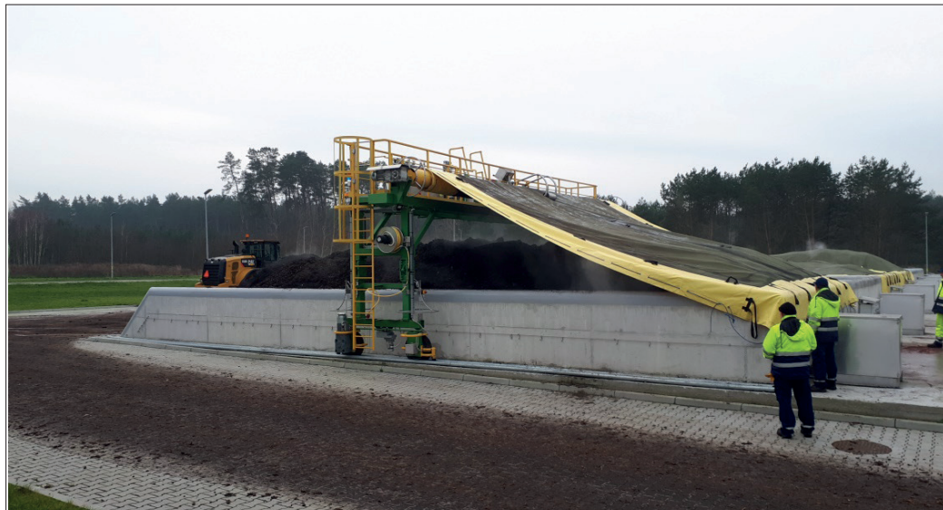
Picture 5. Covering the compost reactor with a semi-permeable membrane.
