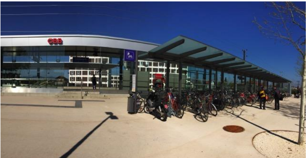
Figure 1 Roofed bicycle parking at Laterach Station, Austria (Photo: Takeru Shibayama)
