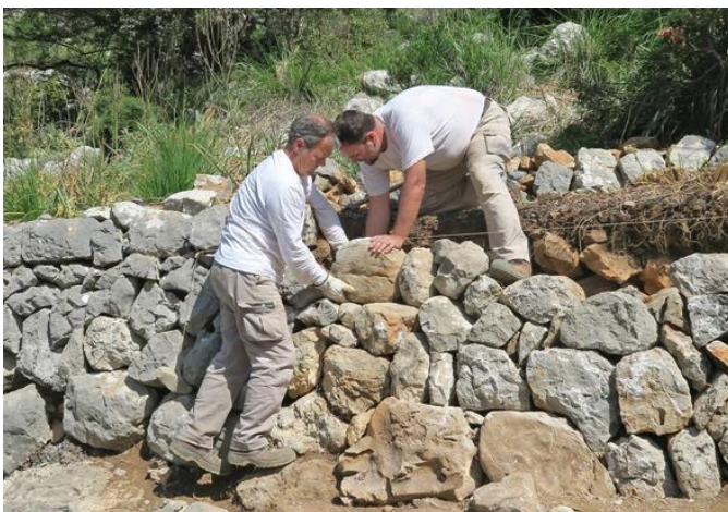
Dry stone recovering works
