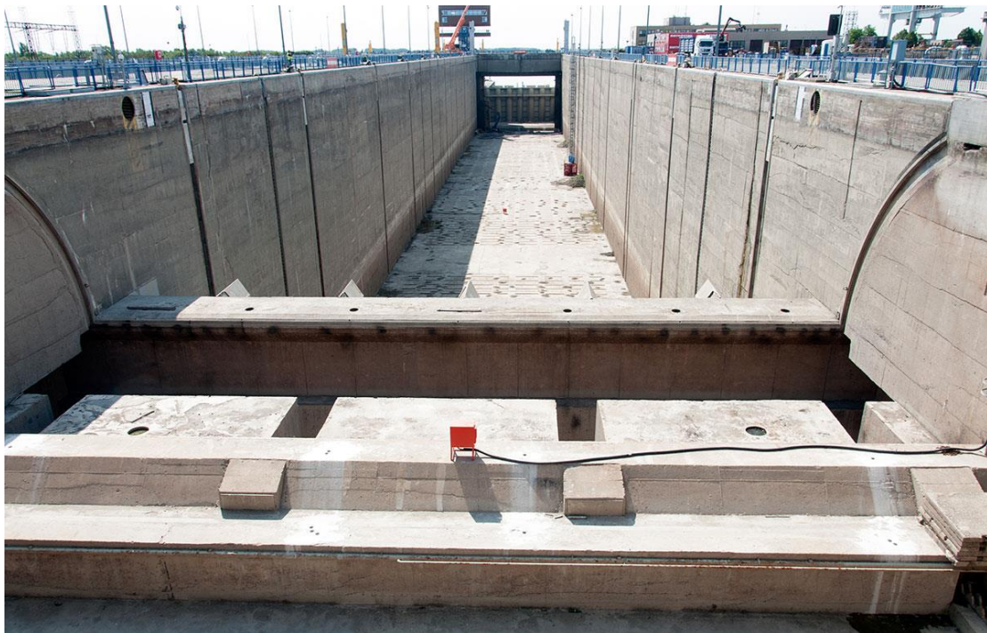
Figure 5 Example of locks restoration - Gabčíkovo
