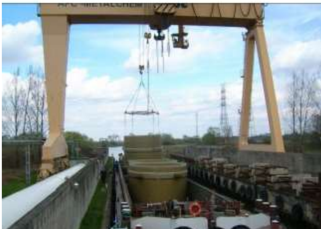
Fig. 1. Unloading of chimney liners, Source: [Fot. Damian Bednarz].
