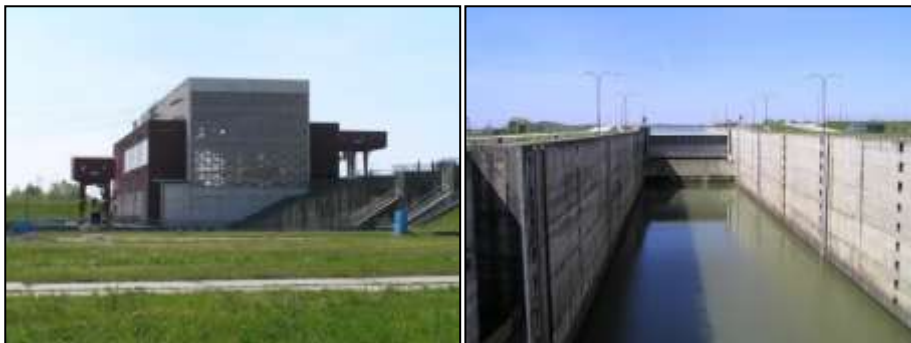
Figure 9 – Waterwork Kráľová and its lock
