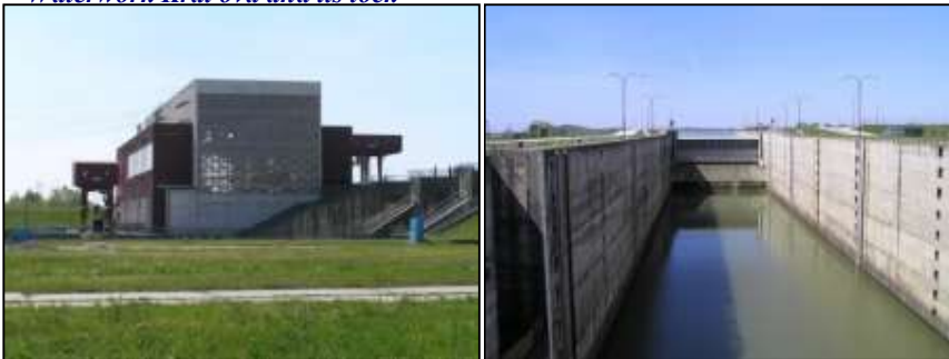
Figure 9 – Waterwork Kráľová and its lock
