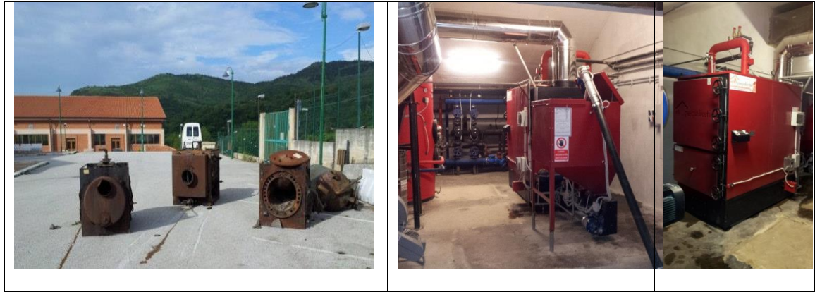
Figure 8 – The decommissioned heating oil boilers (on the left) and the new biomass (pellet) boiler for the swimming pool in the municipality of Petralia Sottana.
