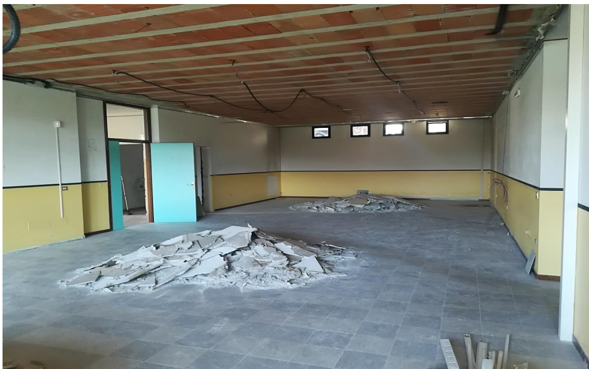
Photo 2 - removal of false ceilings
