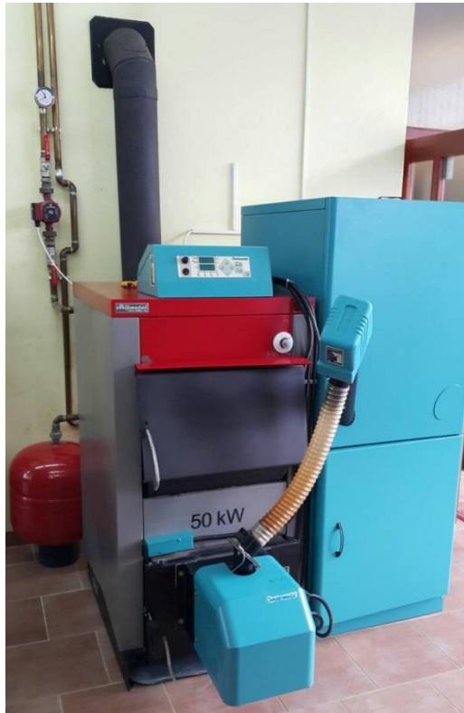
Figure 4. – Pellet furnace 50 kW of power
