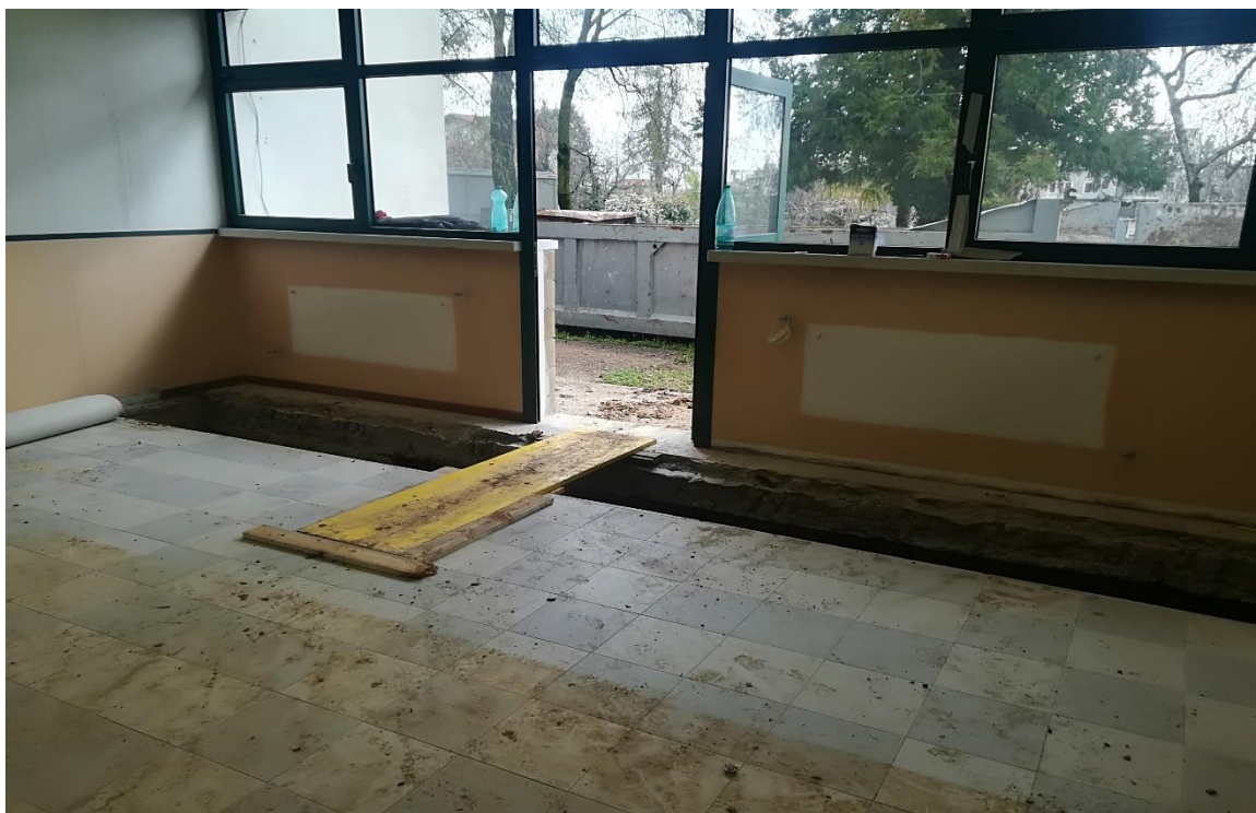
Photo 3 - excavations for the construction of new foundations
