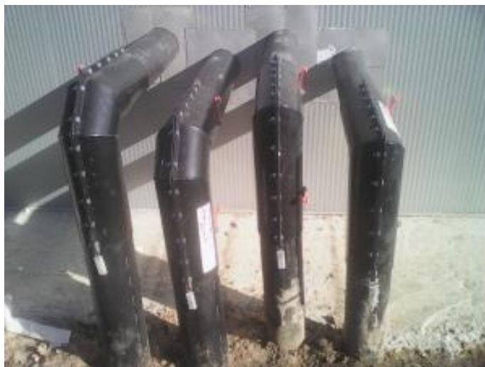
Image 6.4 The four pipes going out of the boiler building.
