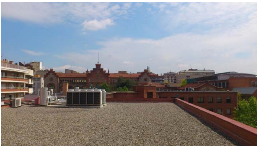
Figure 7 The roof, walls and AC equipment of library
