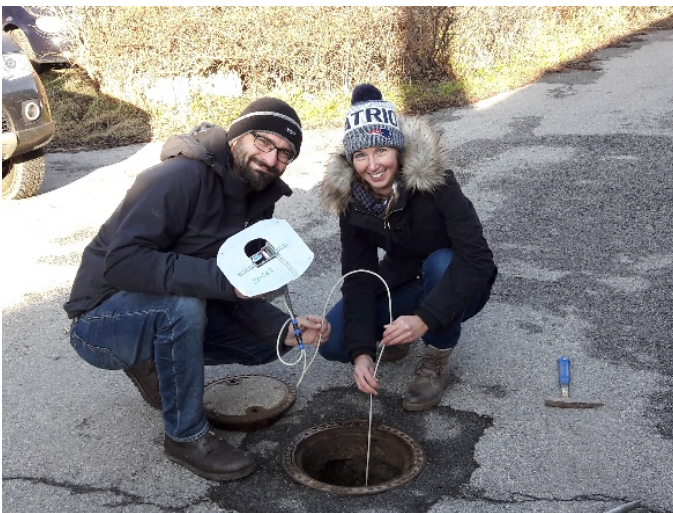
Figure 5. Installation of automatic groundwater temperature logger WTF in low-level observation well.
