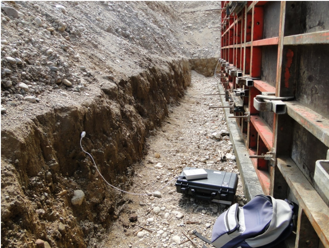
Figure 1: Field measurement of the thermal parameters with the KD2 Pro meter (Janža et al., 2017).
