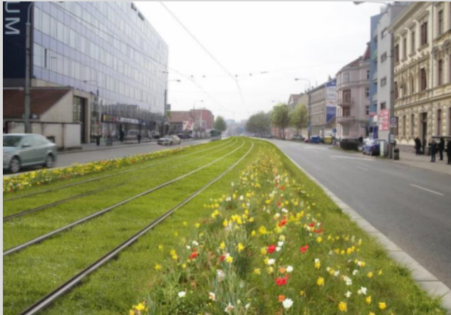
Visualization of reconstruction of tram lines Nové sady where "green belt" - meadow lawn with flowers will be built for less noise and dust. Photos from www.dpmb.cz
