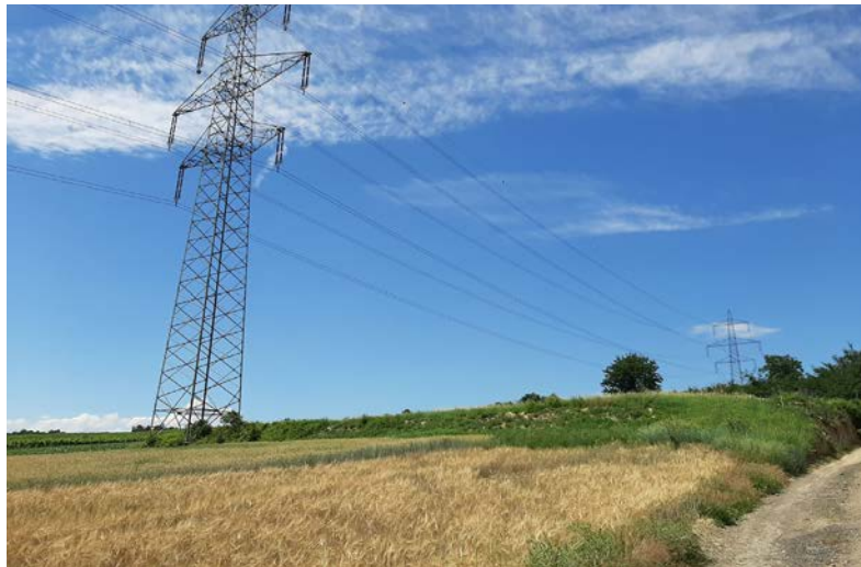
Fig. 3: 380 kV high-voltage power line Dürnrrohr (AT) - Slavětice (CZ)
