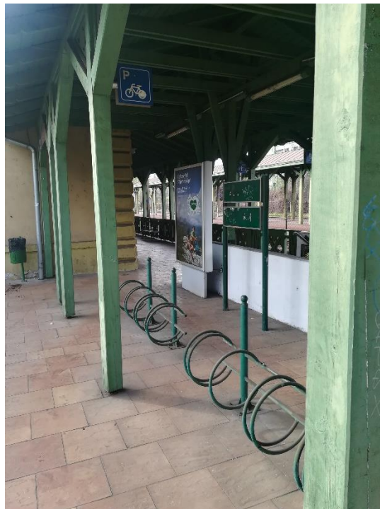
FIGURE 9: B+R STORAGE FACILITIES AT THE RAILWAY STATION PESTSZENTLŐRINC
