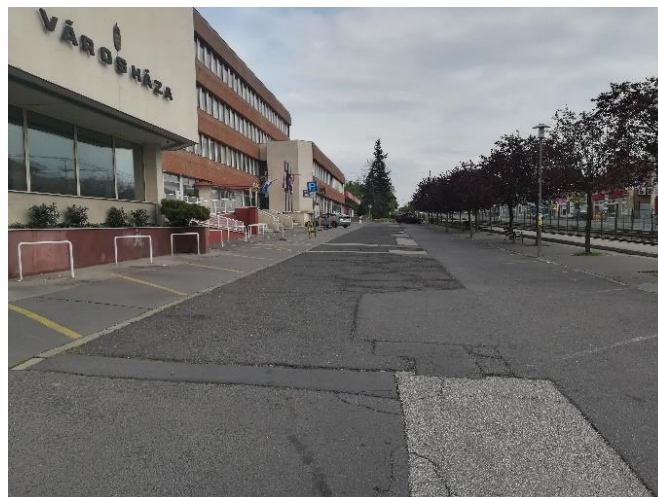
FIGURE 16: THE ENTRANCE OF THE CITY HALL OF DISTRICT 18 WITH A CAR PARK BUT WITHOUT PROPER AND SAFE BICYCLE RACKS
