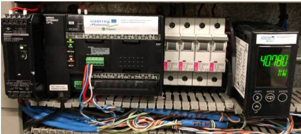
Picture 5: Connection of the measuring equipment into the monitoring system
