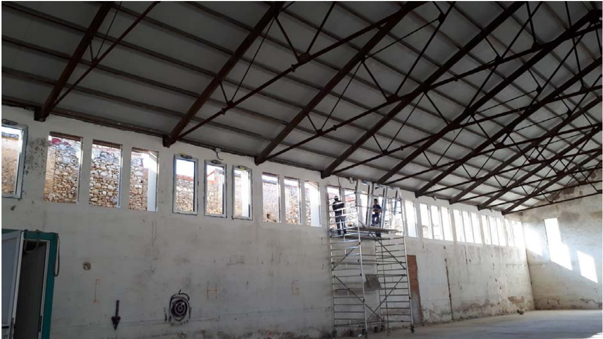
Figure 27 : Mounting new windows (innovative solution) 2
