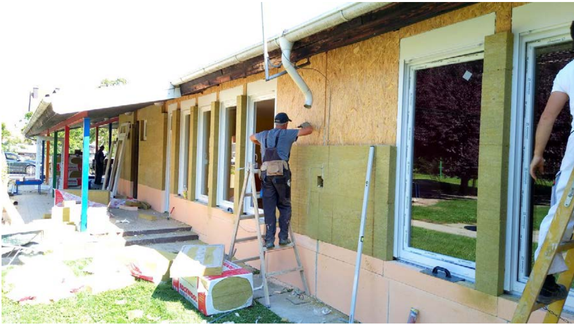
Figure 11 : Mounting the mineral wool
