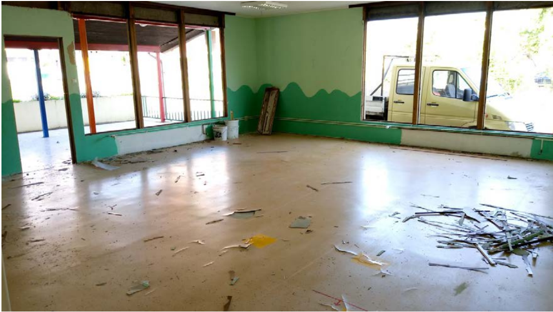
Figure 17 : Children rooms before 1
