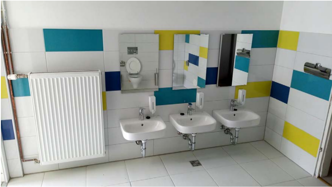
Figure 5 : The bathrooms after the works have been done 1
