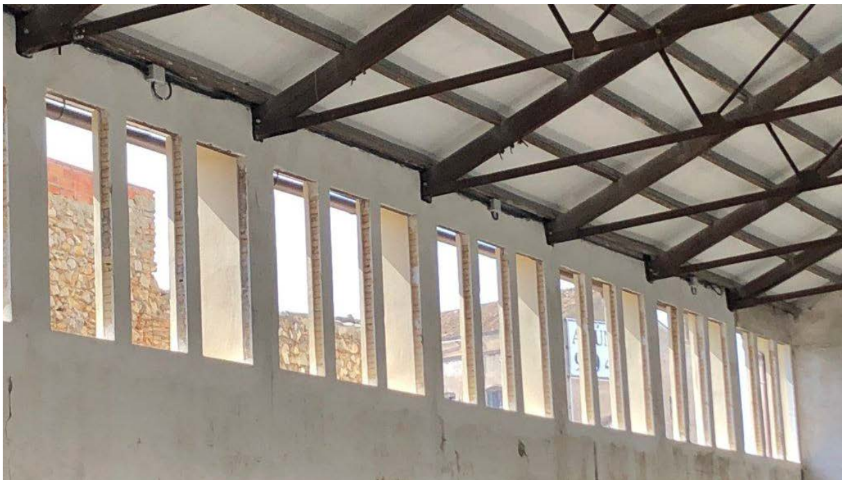
Figure 25 : Old windows removed
