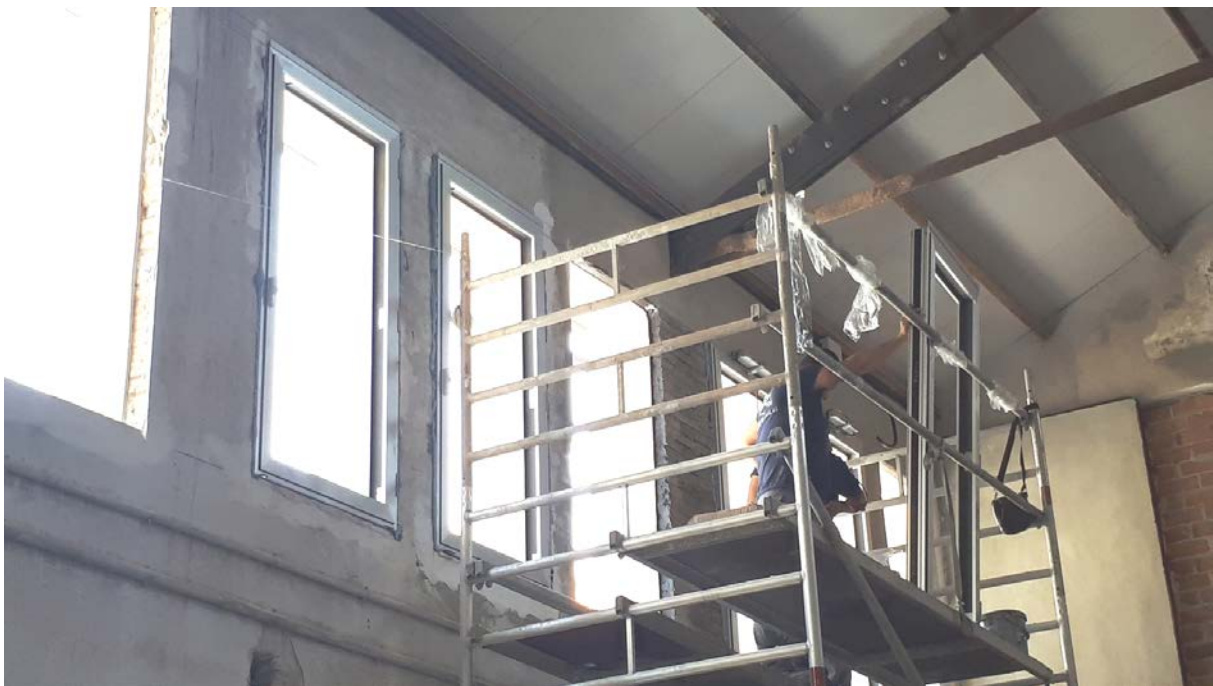
Figure 26 : Mounting new windows (innovative solution) 1
