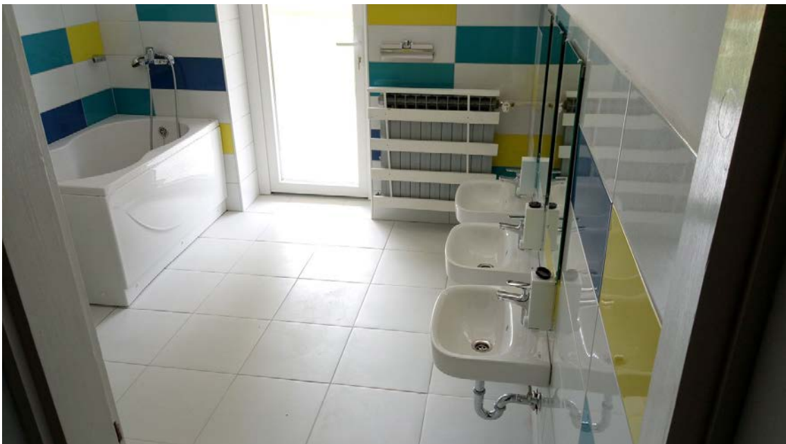
Figure 6 : The bathrooms after the works have been done 2
