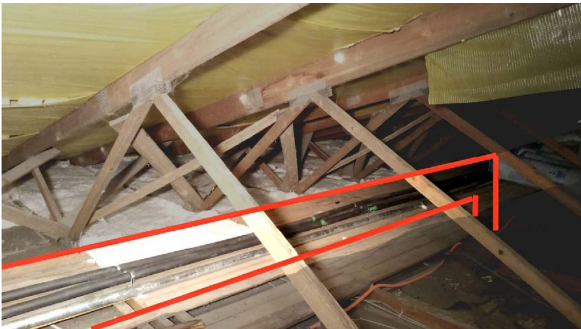
Figure 1 : The attic used for laying down the water supply pipes...
