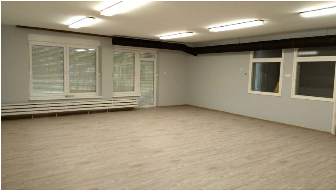
Figure 19 : Children rooms after – new floors, ventilation with recuperation
