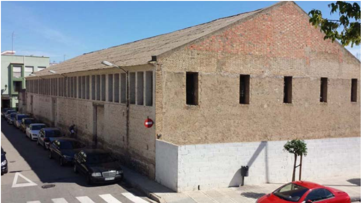
Figure 22 : Magatzem de Cucó exterior view
