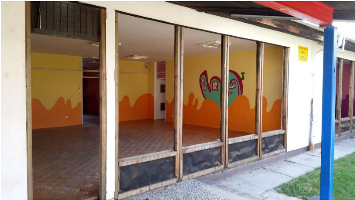
Figure 7 : The original building wooden envelope
