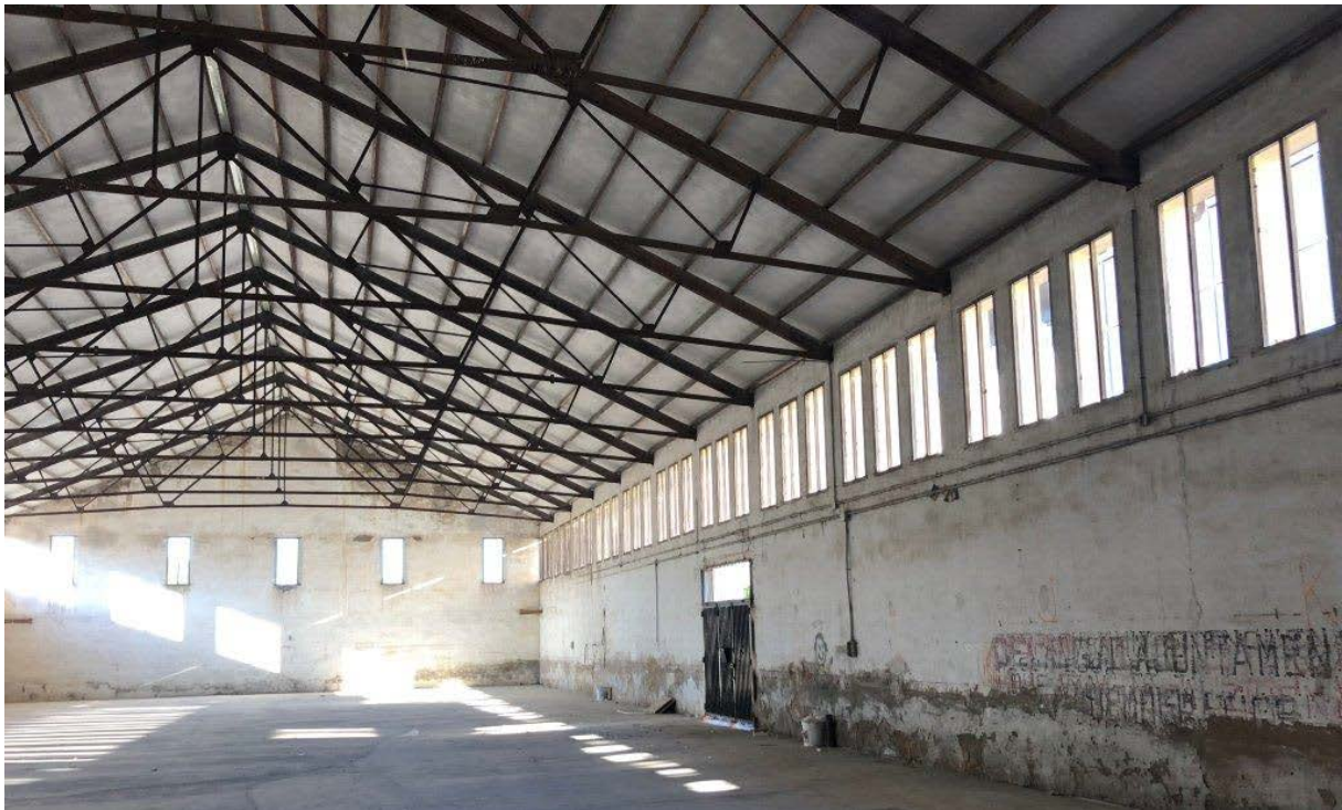
Figure 23 : Magatzem de Cucó interior view
