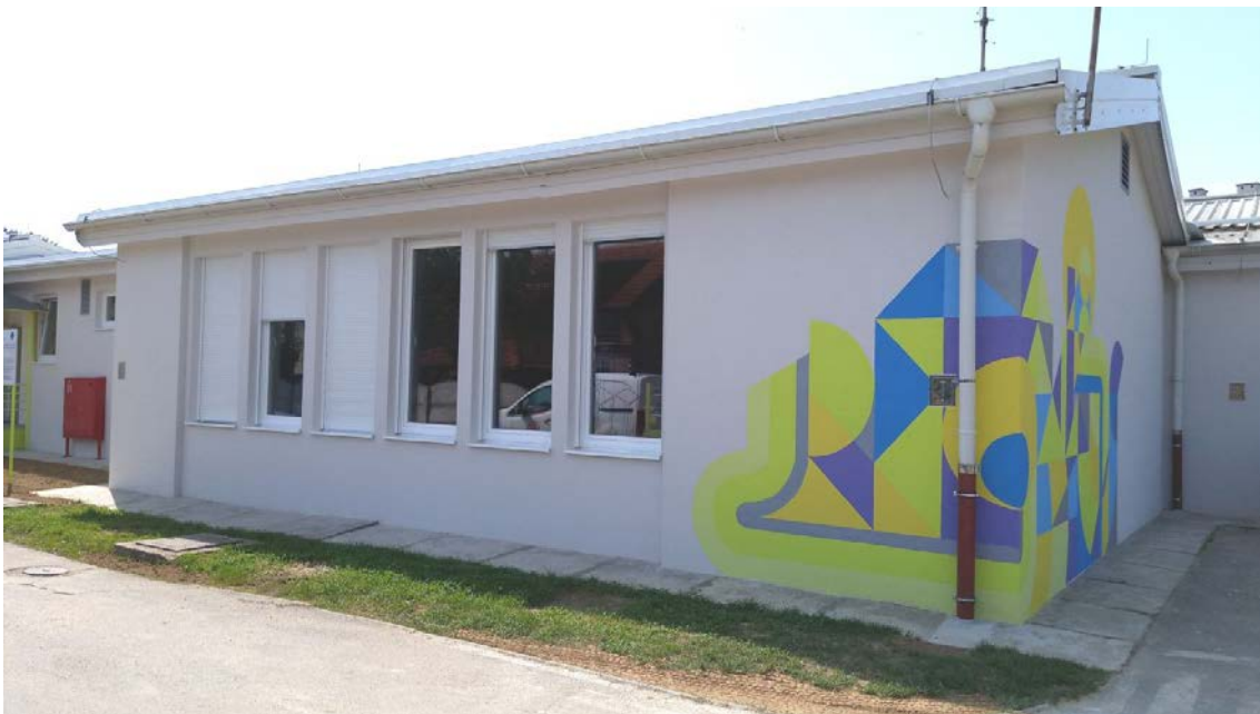
Figure 16 : A new façade and some new pretty drawings
