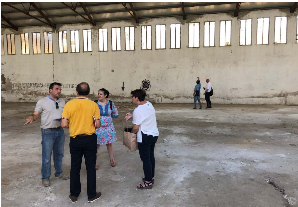
Figure 24 : Windows before works
