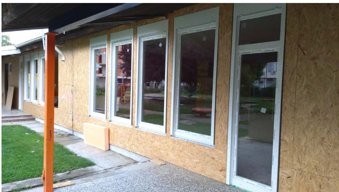
Figure 10 : An envelope after reinforcing
