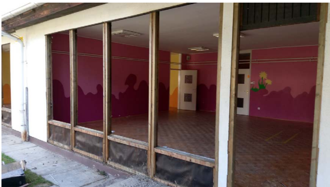
Figure 9 : An envelope before reinforcing
